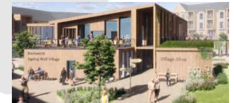
Aging Well Village, Backworth Park, Newcastle-Upon-Tyne
