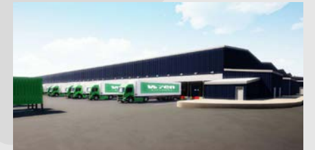
Wren Kitchens New Factory
